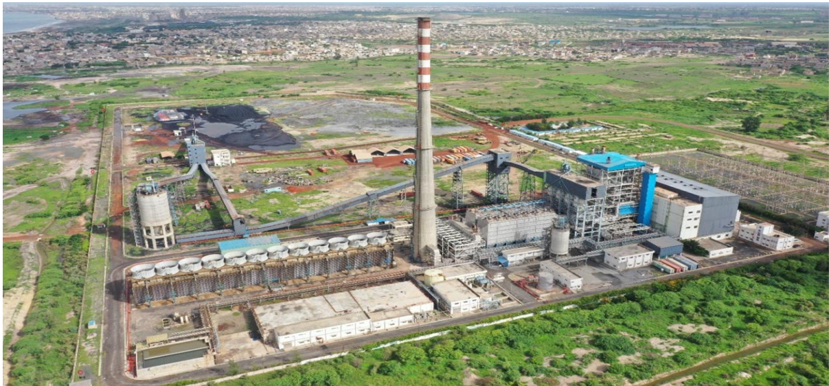
Photo 1. Sendou power plant with coal storage and ash dumping facility facing the city of Bargny. Source: Sebenzana, September 2022.
