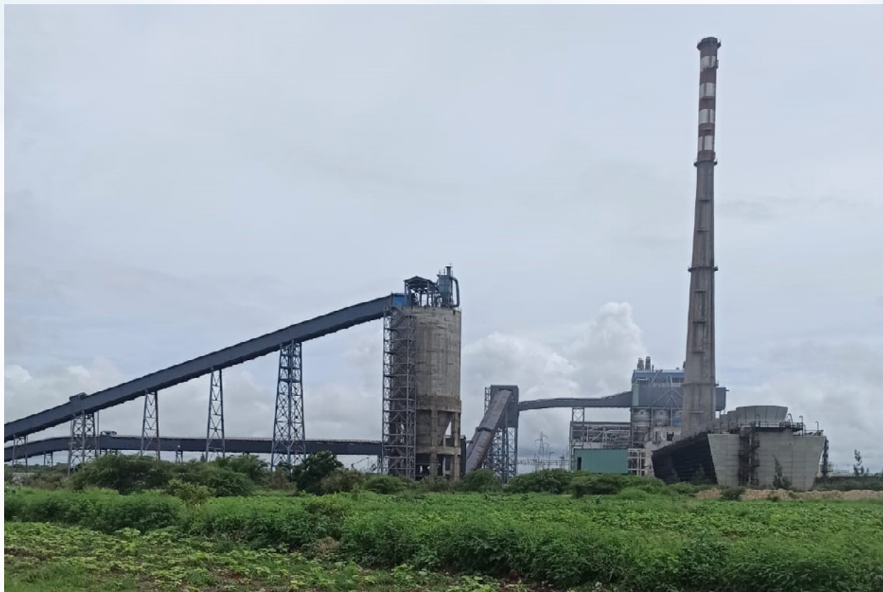
View of the Sendou power station in Senegal, September 2022.
